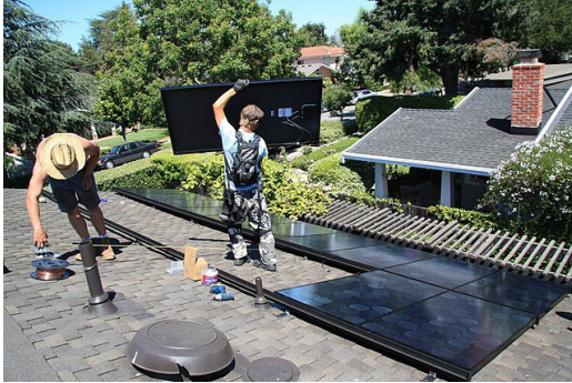
Rooftop solar panel installation
